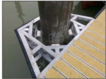
TYPICAL PILE GUIDE
