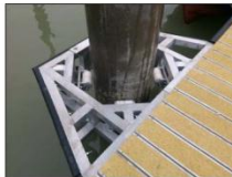
TYPICAL PILE GUIDE
