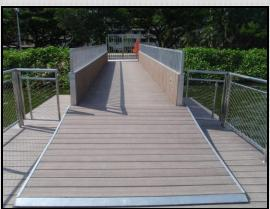
A gangway is an inclined walkway that is connected to an abutment, pier, or bulkhead and supported at the opposite end by a floating structure - usually a transient float.
