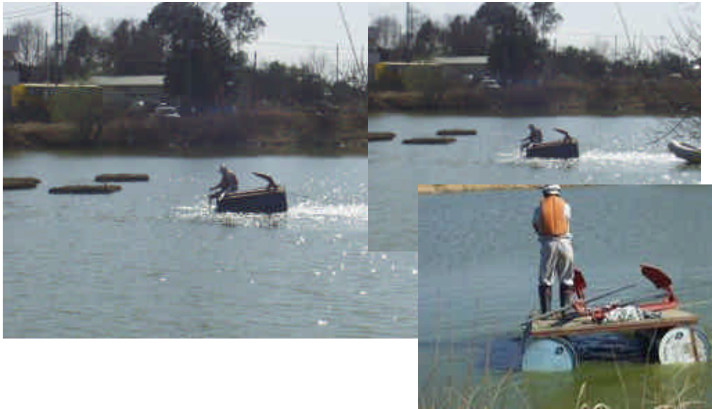
Figure 2-16 Dropping of the anchor
