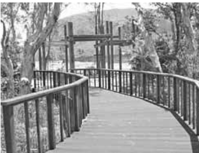
Fig 11 Shelter incorporated into long walk
