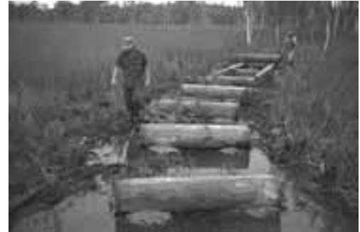
Fig 37 Bedlog installation on poor ground
