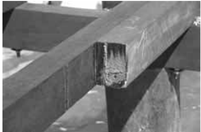
Fig 21 CN Emulsion on cut end
