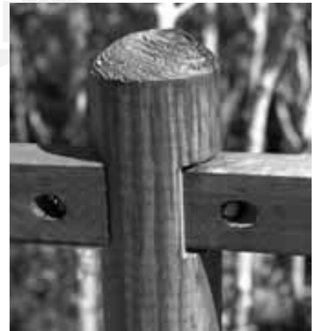
Fig 17 Round handrail post system
