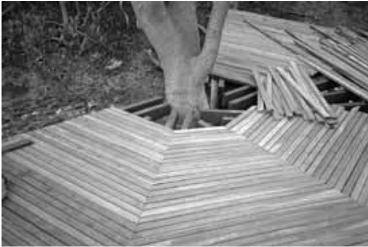
Fig 27 A mitred deck surrounding a specimen tree requires good attention to setting out and experience to achieve a neat result.
