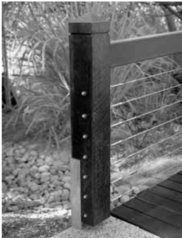
Fig 15 Stainless steel wire as barrier infill.
