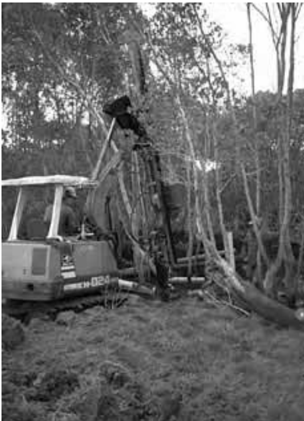
Fig 38 Small pile driver has small footprint
