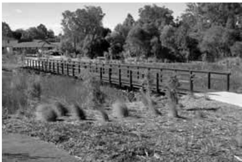
Fig 43 Boardwalk over causeway
