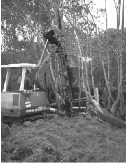
Fig 8. Driving Piles in mangroves
