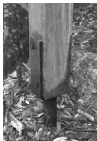
Fig 10 Rock baseplate in cored hole
