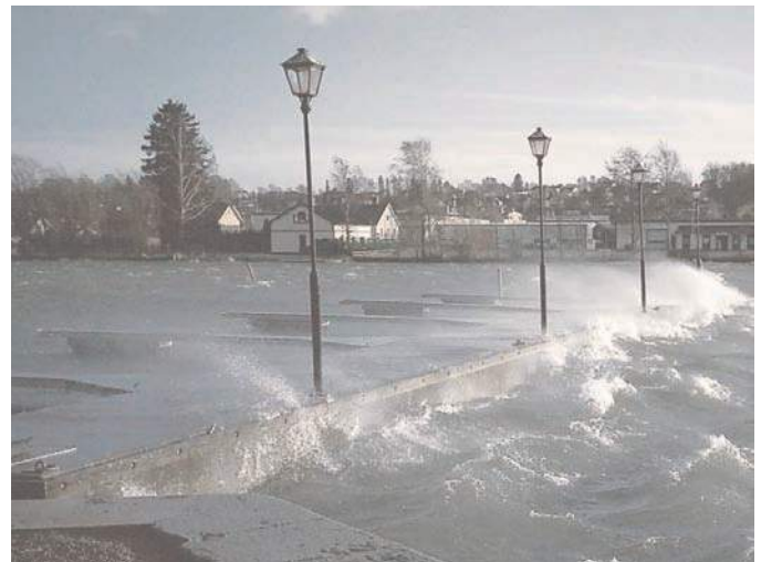
Waves interrupted by a floating attenuator
