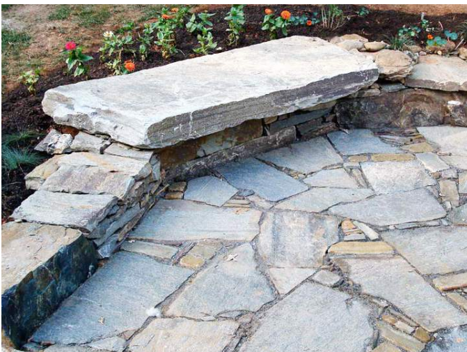
Typical site wall character
