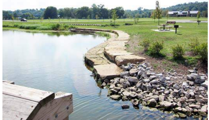
Stacked stone treatment adjacent to typical revetted edge
