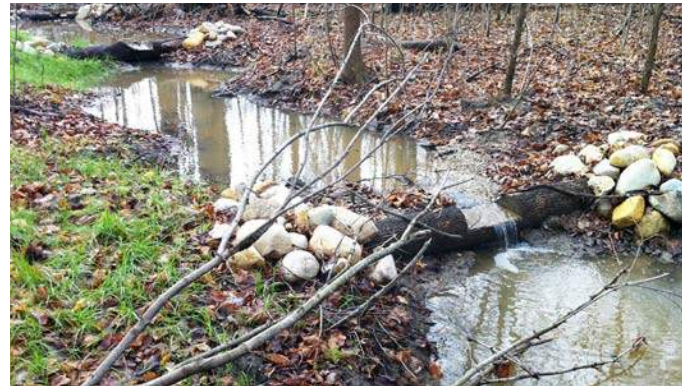
Examples of structures to reduce scour
