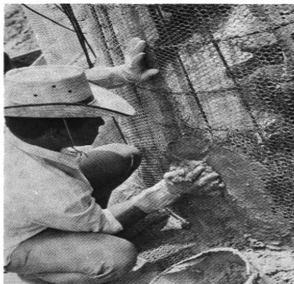
Figure 2.7 A paste of mortar is forced into the layers of mesh by hand
