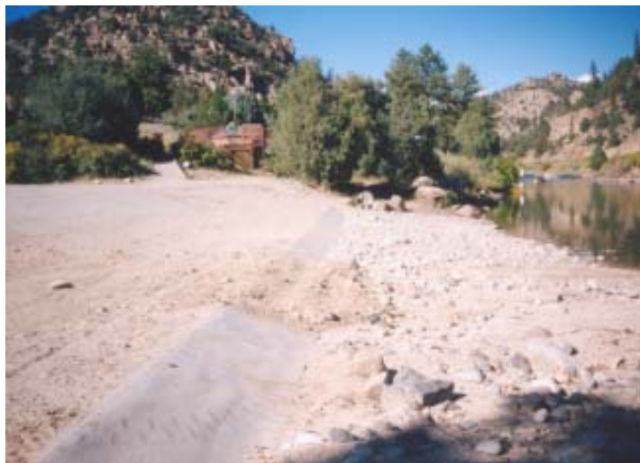
Photo 8M: Concrete strip helps to divert flows away from launch site
