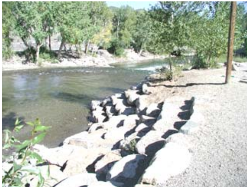
Photo 4G: Restored bank with rock outcrops enables access at varying water levels
