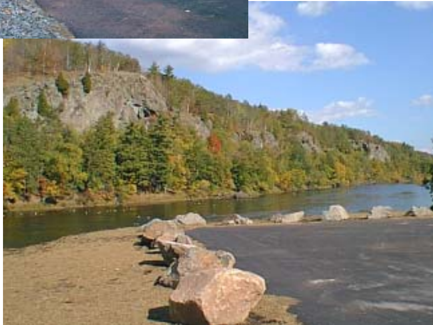
Photo 10D: Little Quinnesec Falls launch area, reinforced with fractured rock riprap
