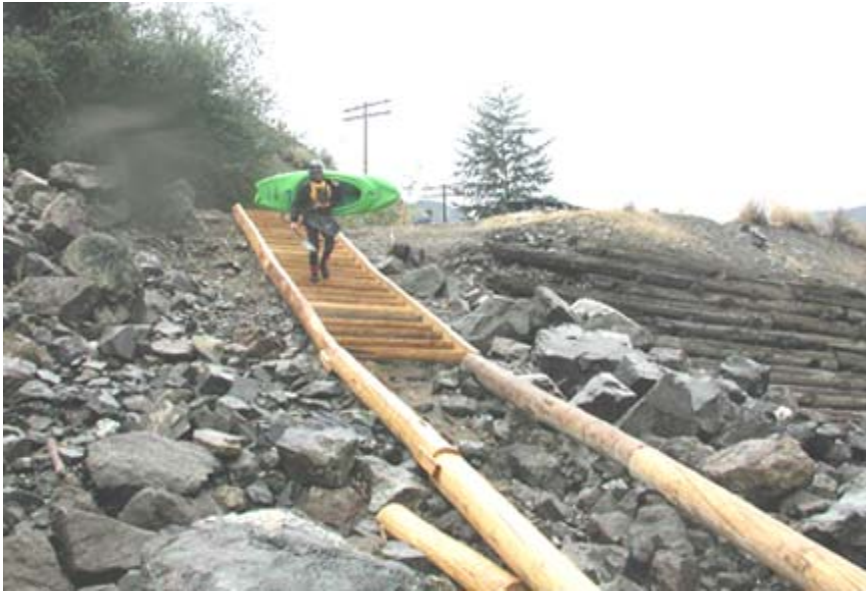
Photo 9E: Rounded timbers serve as staircase for paddlers
