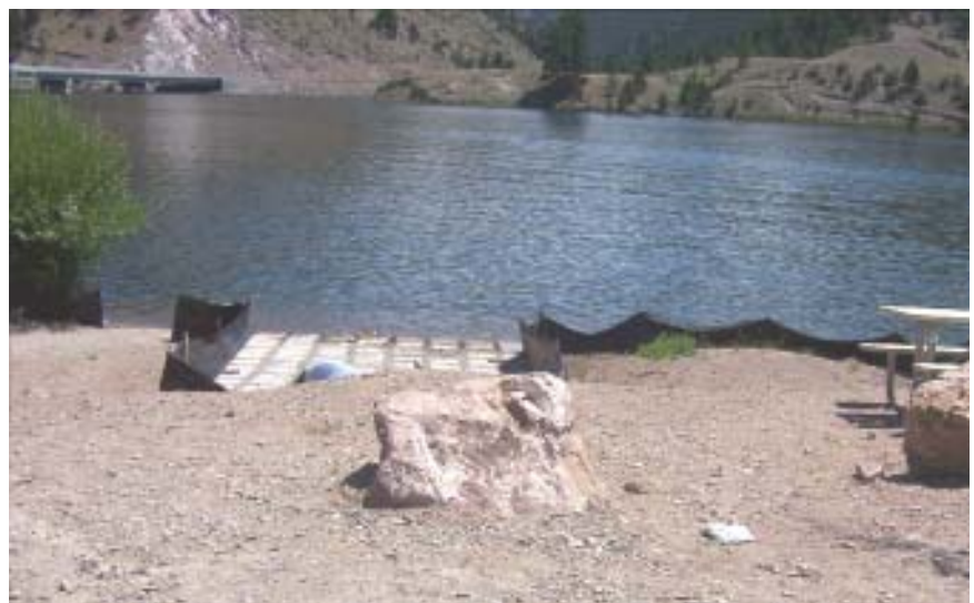
Photo 8I: Articulated concrete launch helps to mitigate erosion while providing paddlers with a separate access site from heavy boat traffic
