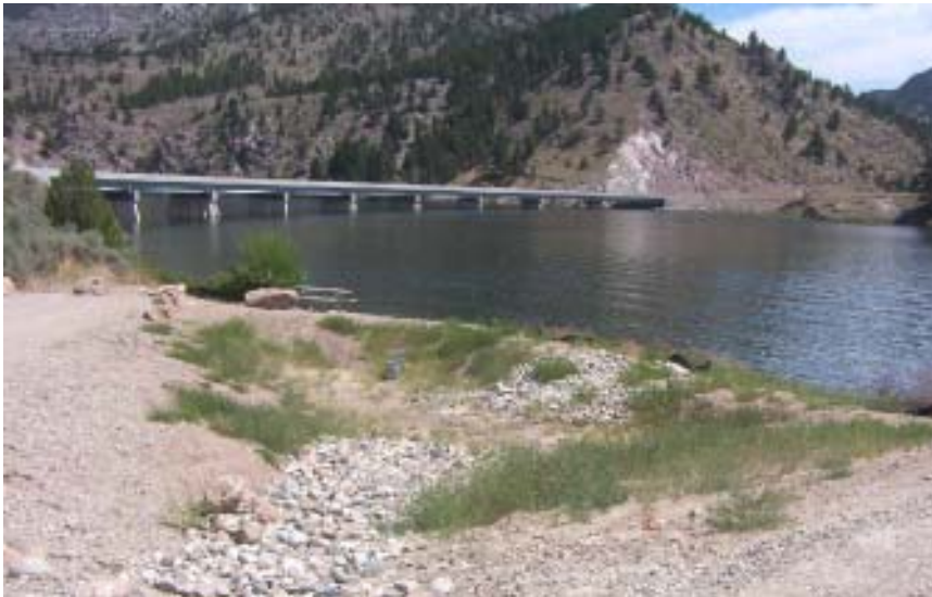
Photo 8H: Gravel road provides access to both the launching area and a detention basin used for maintenance purposes
