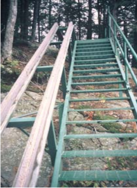
Photo 10F: Detail of metal staircase, wooden boat slide, and handrail
