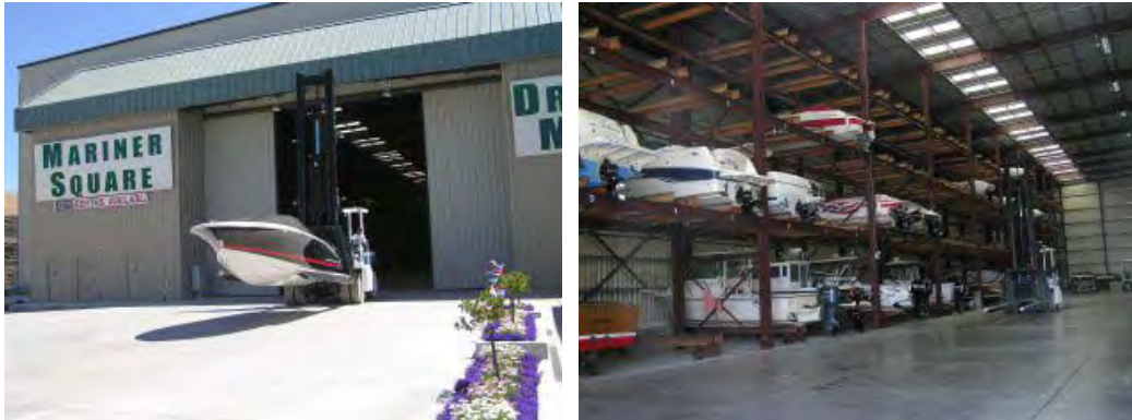
Figure 8-3, Drystack (rack) Storage
