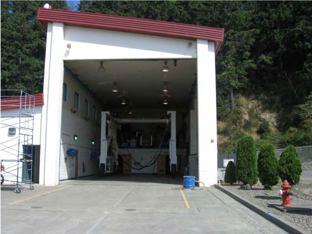
Figure 9-2, Enclosed Shop Building, with Straddle Carrier
