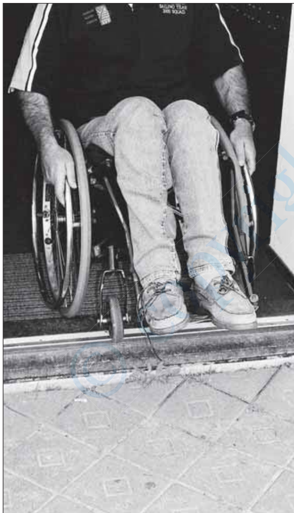
Pic. 2: Obstruction in the path of travel
