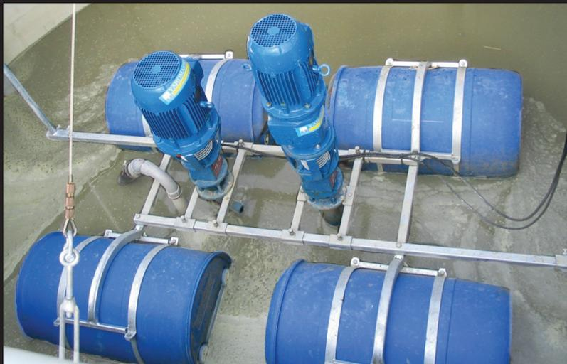
In smaller tanks there is a vertical guide system which also supports the pontoon when pumping out.
