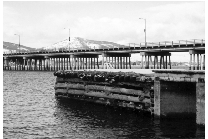
Figure 11—This aging crib dock continues to provide sturdy recreation access in a lake that is subject to icy conditions.
