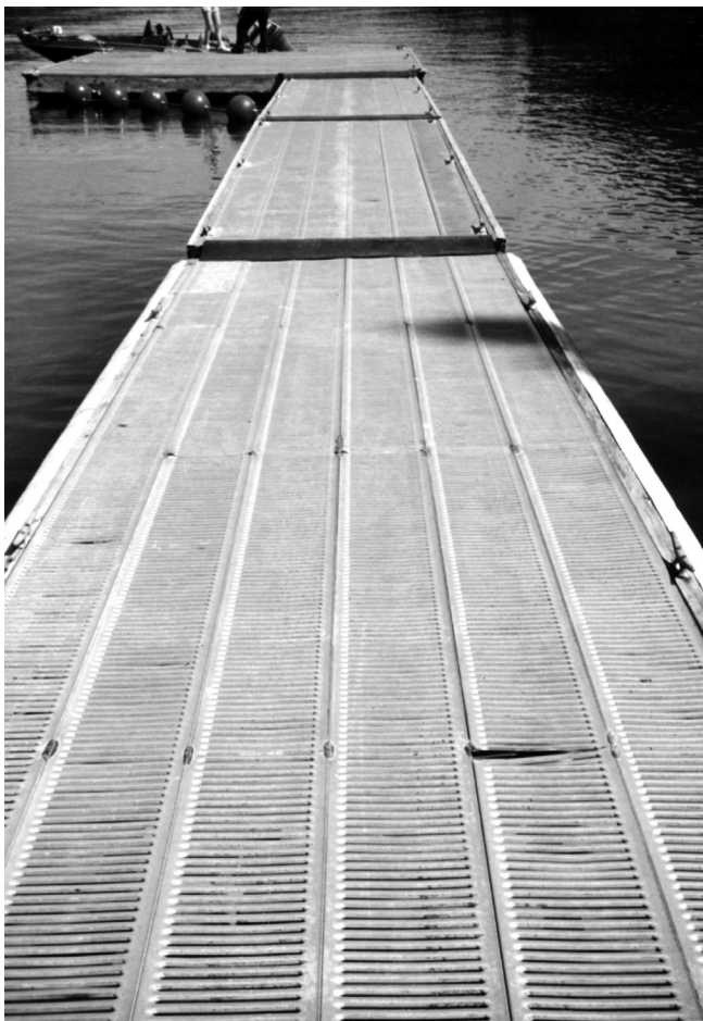
Figure 4—This dock at Dworshak Reservoir in Idaho uses metal grating as its deck. Metal decking provides drainage and traction but can still be slick when it is muddy and wet.
