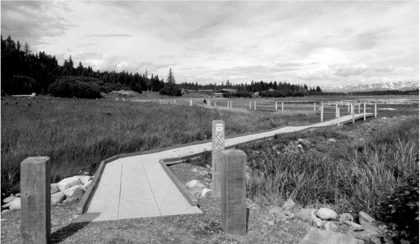
Figure 8—This floating bridge crossing a wetland in Alaska uses the Superdeck modular system (photo by Paul Schrooten, USDI Fish and Wildlife Service).
