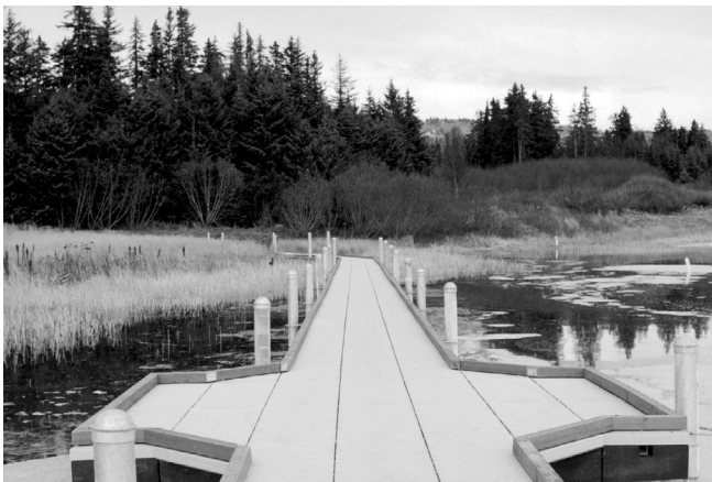
Figure 15—Side extensions to this floating trail bridge provide places where users can stop without obstructing others (photo by Paul Schrooten, USDI Fish and Wildlife Service).
