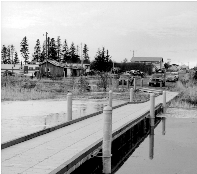
Figure 22—This dock uses multiple external pile holders for anchorage (photo by Paul Schrooten, USDI Fish and Wildlife Service).
