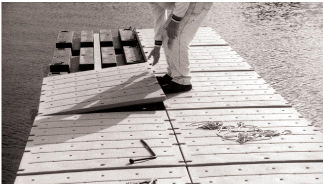
Figure 1—This commercially available modular dock system is easily assembled using common tools (photo by Paul Schrooten, USDI Fish and Wildlife Service).
