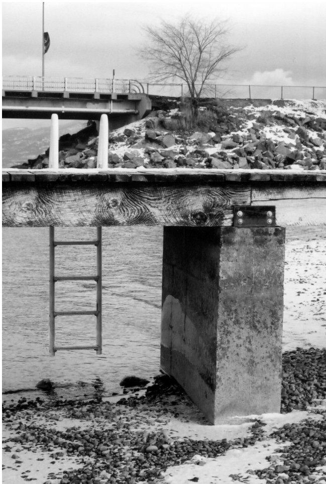
Figure 6—A concrete support makes an excellent foundation.
