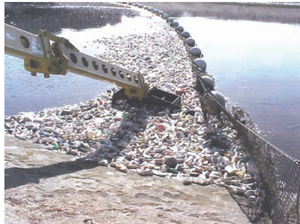
Figure 3. Los Angeles River litter boom system (courtesy of Los Angeles Department of Public Works).
