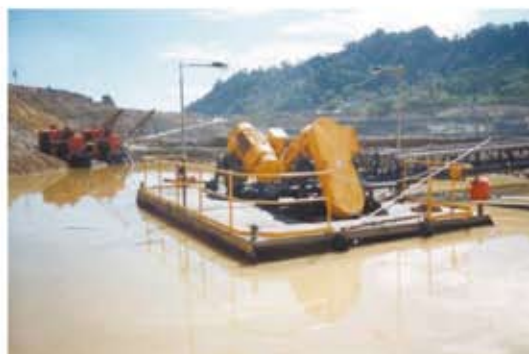
Left: A double pontoon pump unit operating in high temperature, low pH, high solids content water at a mine in Papua New Guinea.
