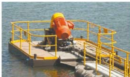
Left: A single ME unit with floating walkway operating at a process plant in Indonesia.
