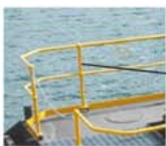
Hand railing including kick rails
